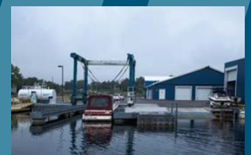
50 Ton Lift | Launch Ramp
